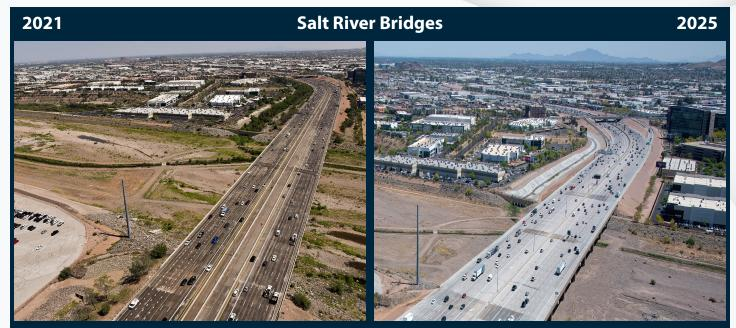
Crews widened the I-10 bridges over the Salt River to make room for six general purpose lanes and two HOV lanes in both directions.
