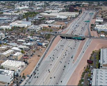
Crews reconfigured the I-10 interchanges at 32nd and 40th streets, which included removing the loop ramp that connected southbound 40th Street to eastbound I-10.
