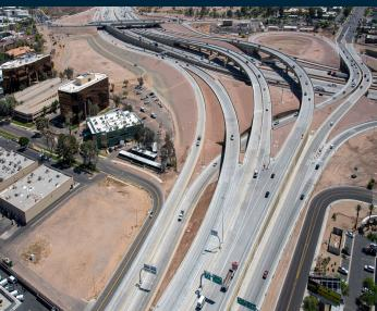
Crews rebuilt the I-10 interchange with SR 143 to improve traffic flow and create direct connections to and from SR 143 for drivers in the I-10 HOV lanes.
