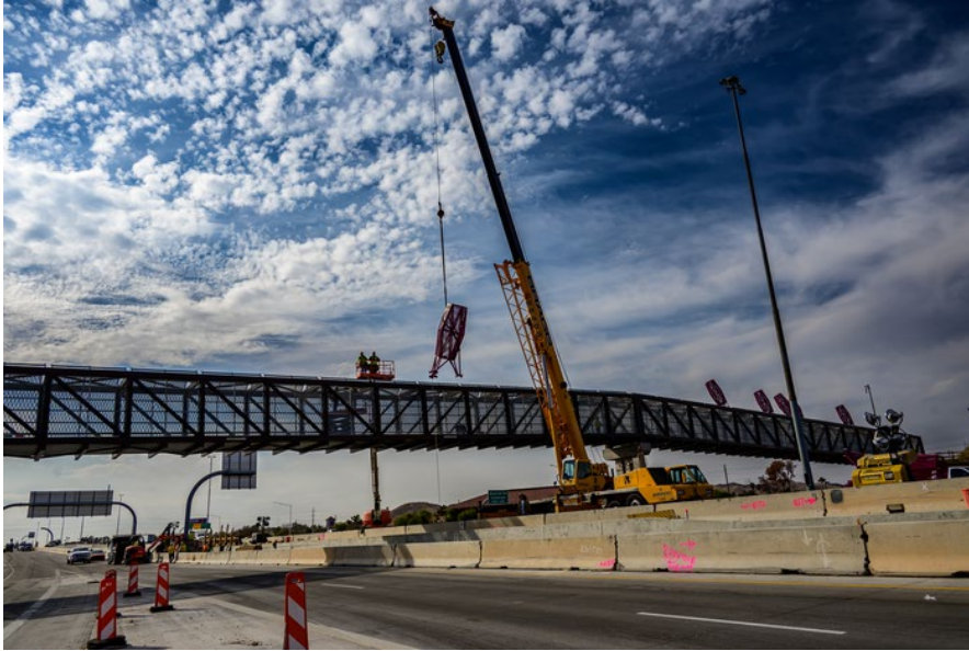
A crane lifts one of the decorative pieces onto the multiuse bridge at the Western Canal.
