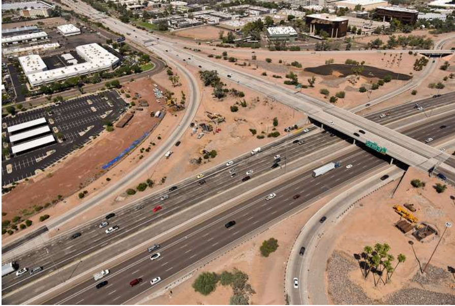
The SR 143 and I-10 interchange in 2021.
