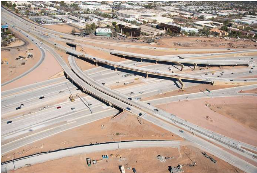
The SR 143 and I-10 interchange in 2024.
