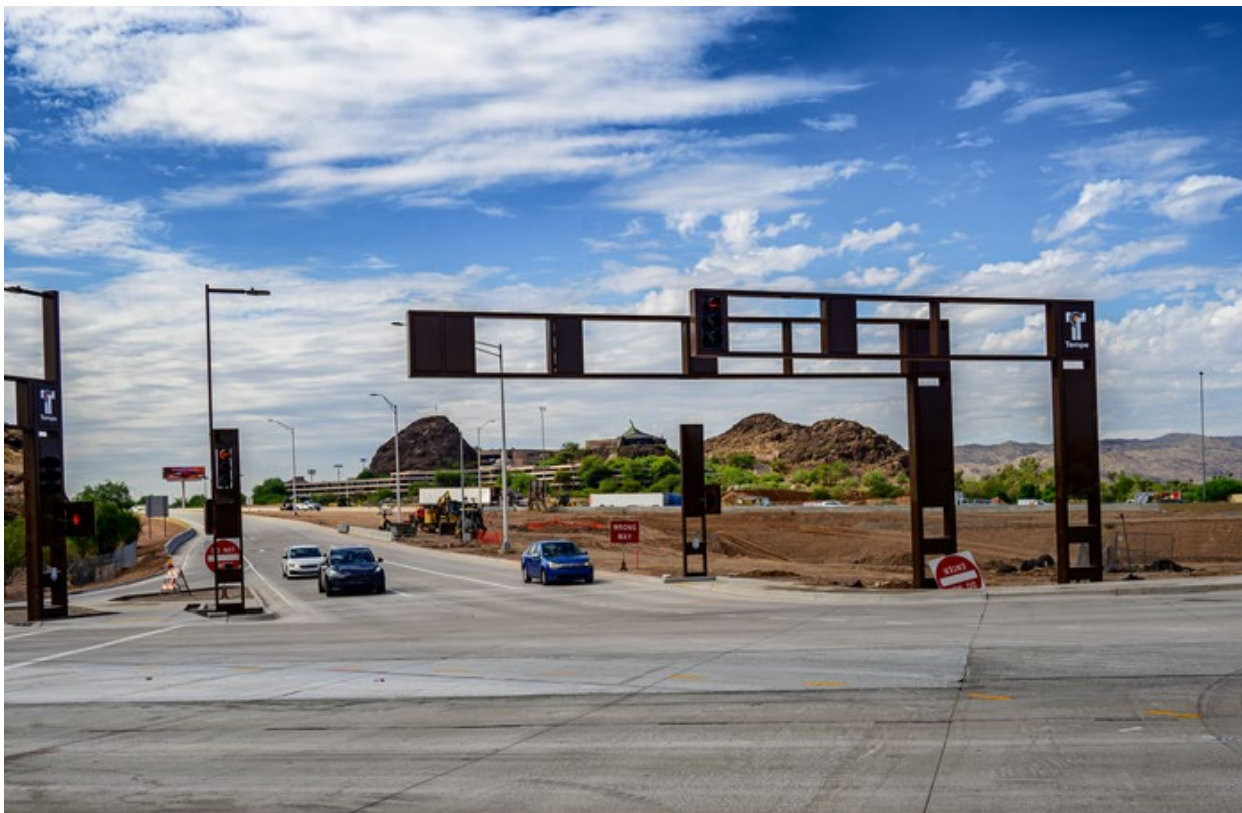
The westbound I-10 off-ramp at Broadway Road reopened August 26.
