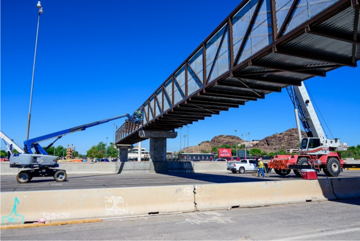
Crews installing fencing on the multiuse bridge at Alameda Drive.
