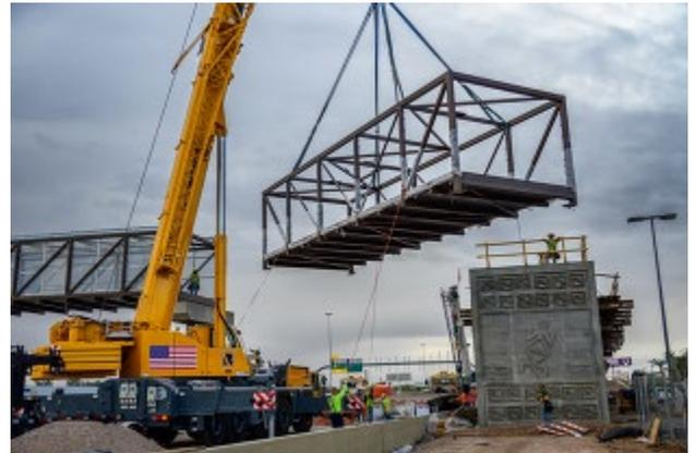
*In the photo above, a crane lifts the piece of truss that will connect the multiuse bridge over I-10 to the west-side landing at Alameda Drive.*
