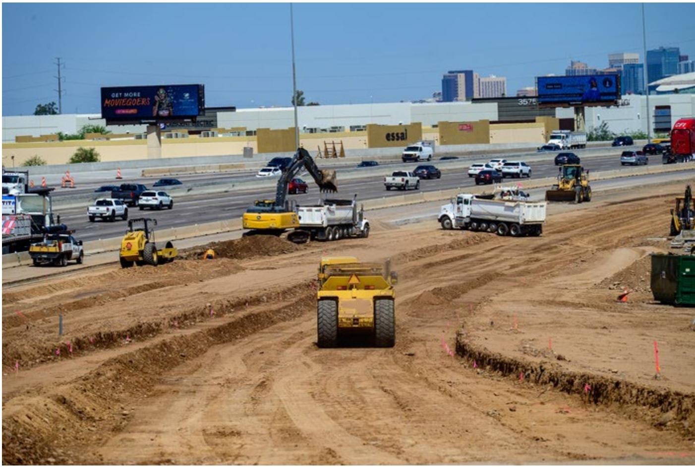
The westbound I-10 on-ramp at 32nd Street is closed for reconstruction into September. Crews are currently doing the earthwork necessary to reconstruct the ramp. Drivers should use the westbound I-10 on-ramp at 40th Street as a detour during this closure.
