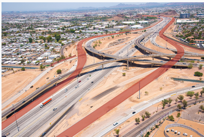
The CD roads, highlighted in red, collect traffic from the I-10 mainline, SR 143 and US 60 and distribute it to crossroads or other highways.
