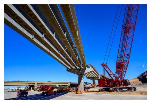
These girders will form the support for the bridge deck of the ramp connecting southbound SR 143 to eastbound I-10.
