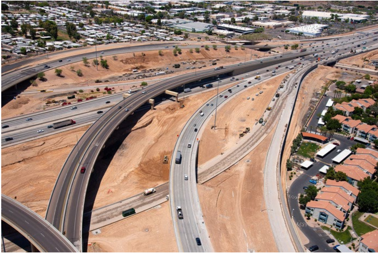
Shown here are the HOV lanes connecting US 60 and I-10.
