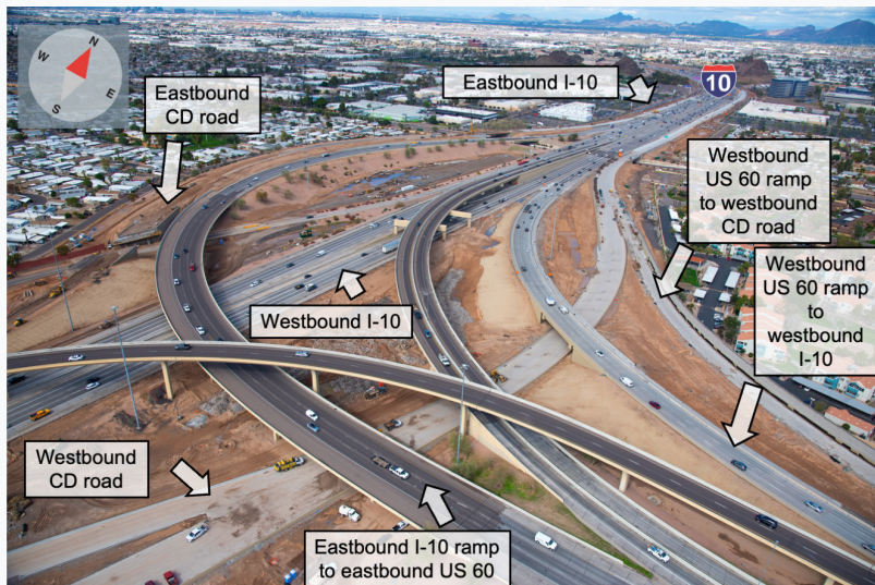
When complete, the CD roads will collect traffic from the I-10 mainline, SR 143 and US 60 and distribute it to crossroads or other highways.
