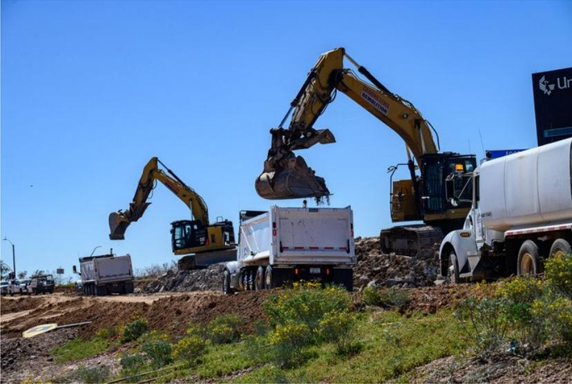
*Crews break up and remove the pavement that used to be the eastbound I-10 off-ramp at 32nd Street.*
