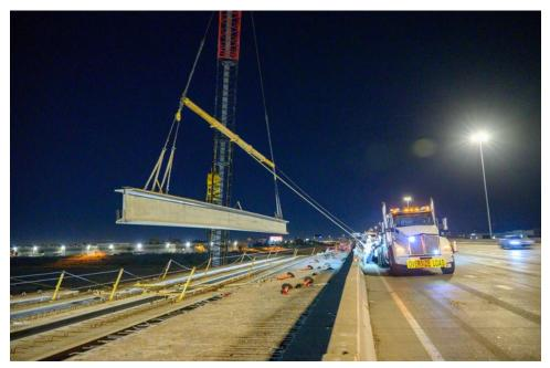
A crane lifts a girder from westbound I-10 at the Salt River and slowly moves it into position on the new bridge caps.
