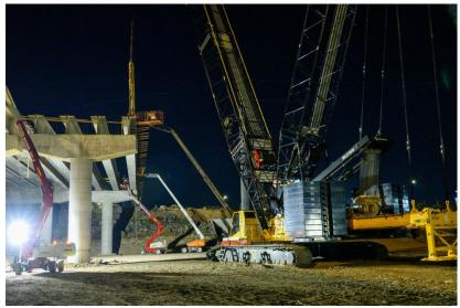
Once the girder is set, crews then make sure it is stable and secure before disconnecting it from the crane.
