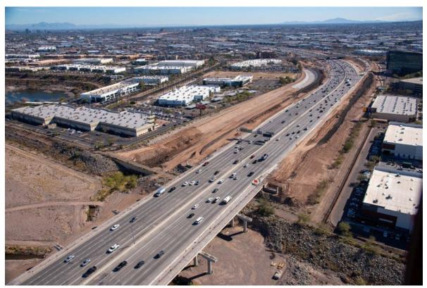
Crews are replacing the lining of the Tempe Drain along westbound I-10 between 32nd and the Salt River with a concrete liner to reduce future maintenance needs.
