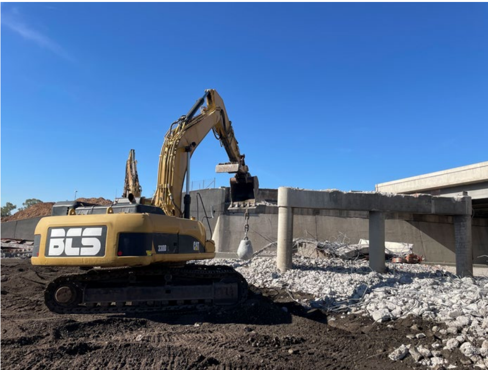
A crew removes the old 48th Street bridges over I-10.
