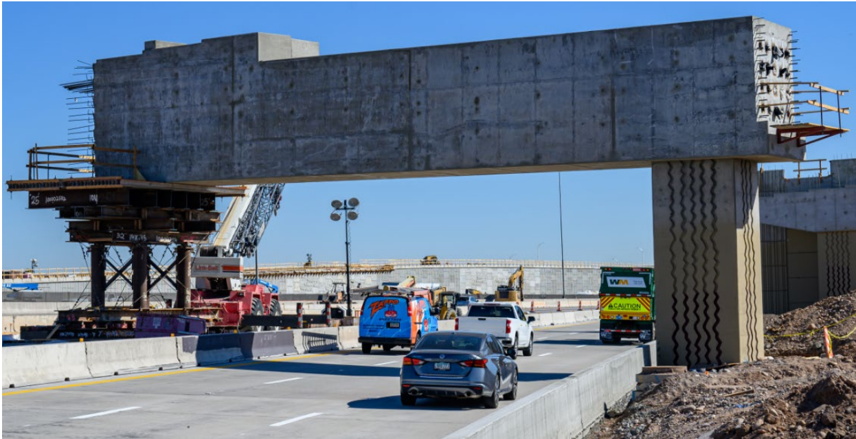
Eastbound I-10 motorists drive under a partially built straddle bent between 48th Street and Broadway Road.
