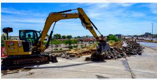
Workers remove the westbound I-10 off-ramp at 40th Street pavement to reconfigure the ramp and make room to widen I-10.
