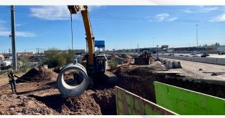
As part of the ramp reconfiguration, crews relocate storm drain pipe under the westbound I-10 off-ramp at 32nd Street.
