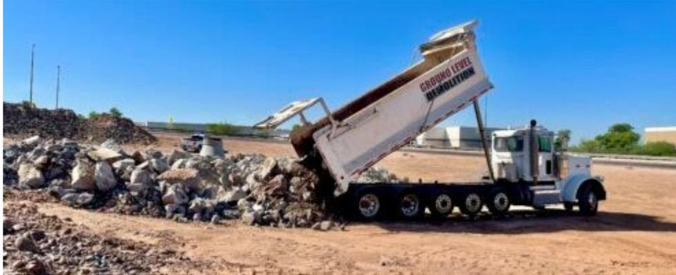
This concrete debris will be broken up into smaller pieces and used for embankments or as fill to build up approaches for new bridges.
