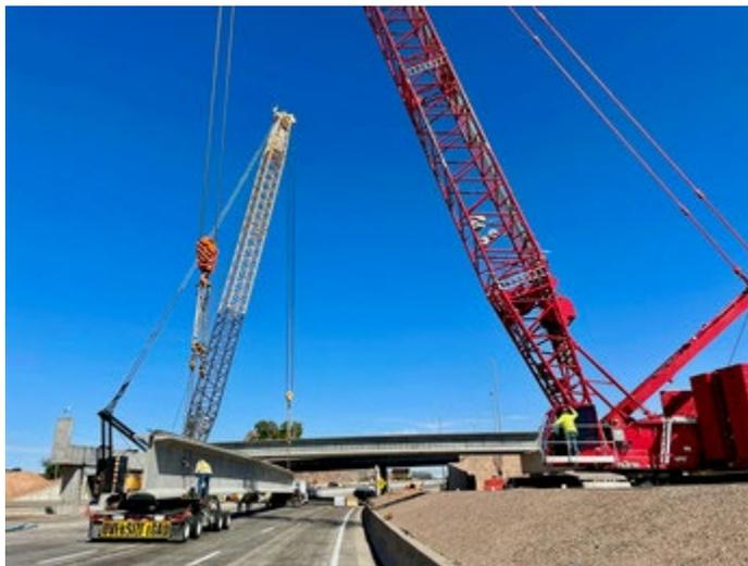
**Decks on Deck:** Construction of the new 48th Street and Broadway Road bridges over I-10 will also continue during phase two. In June and early July, crews successfully set the girders for both bridges, and are now preparing them for their decks (the part you will drive across). Placement of the new 48th Street bridge decks is set to begin later this summer.
