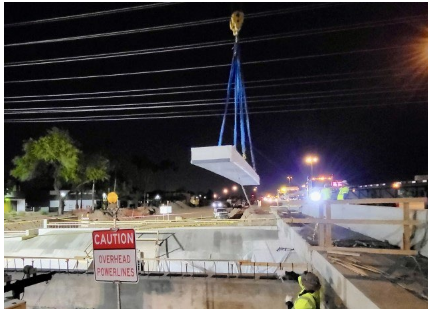
A box beam weighing nearly 40,000 pounds is placed over the Tempe Drain.
