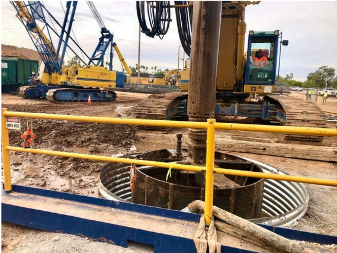
*In January, workers continued installing the drilled-shaft foundations for the new 48th Street bridges over I-10.*
